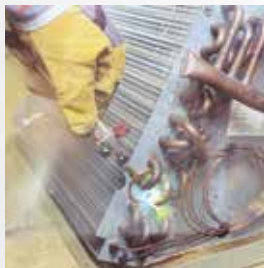
Twin flame tips solder coil return bends quickly and evenly; concentrated heat will not heat and loosen surrounding joints.
